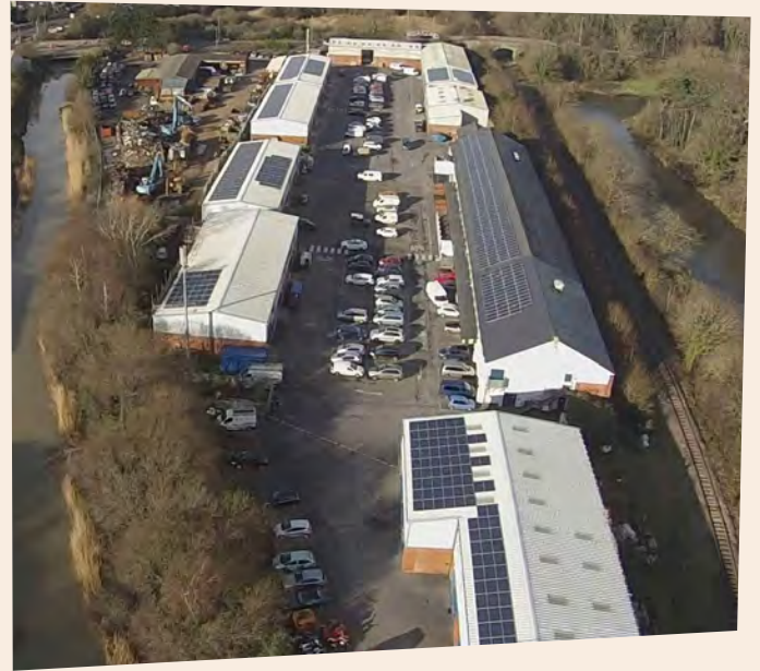
BAPV on industrial roofs at the Olympus Business Park in Newton Abbot. Standard sets of solar panels with metal frames have been used on a low pitch industrial roof. As the setting is industrial, the potential for negative visual impact is low.
