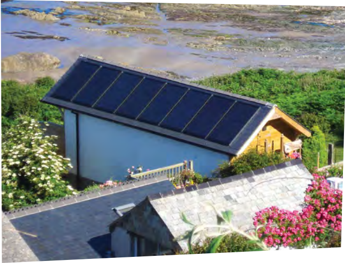
BIPV installation on building in rural Cornwall. The panels are installed to span from eaves to ridge.
