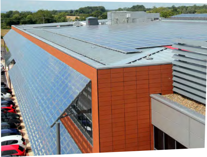
The size of the panels of this brise-soleil matches the size of the tiles on the building's walls (see the case studies section).
