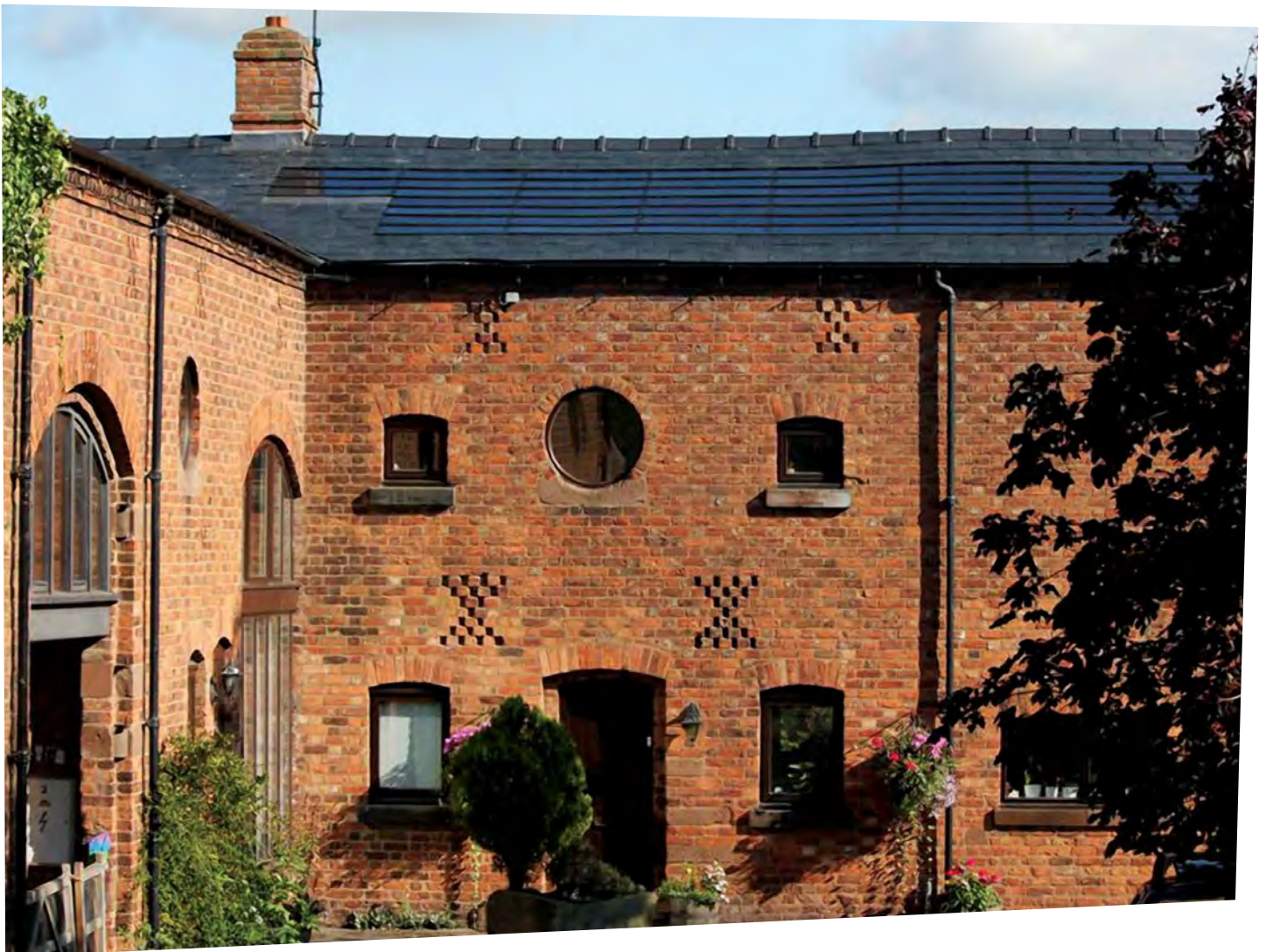
Solar installation and domestic conversion on a listed barn in Chester, installed by The Greener Group.
