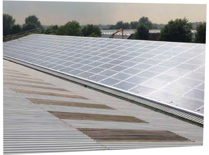
Symmetrical positioning of solar PV on roof valley, covering a roof in its totality.
