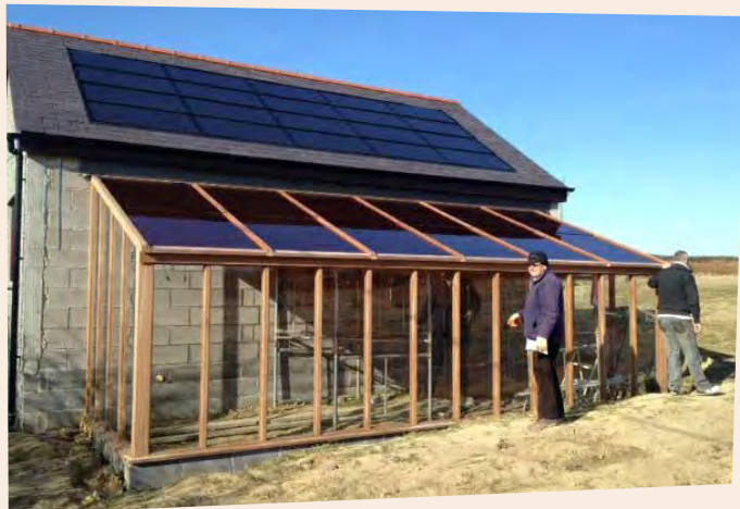
Both images show examples of solar glazing, with different levels of light transmittance. Solar glazing can now be designed into buildings as a form of BIPV.
