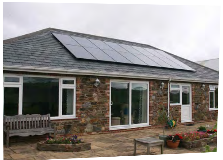
Domestic BAPV installation with frameless panels.
