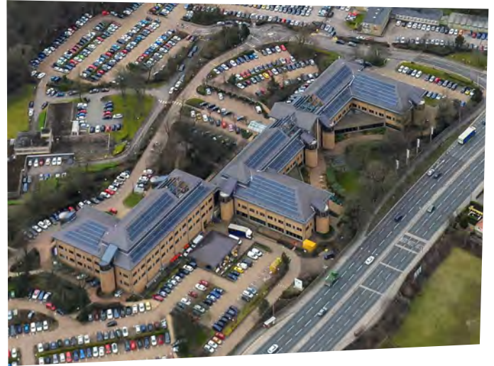
The BAPV installation on Yorkshire Building Society in Bradford demonstrates careful design and implementation of a large solar PV system over a complex, non-symmetrical roof layout.
