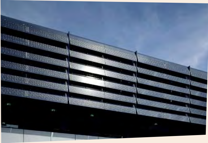
Solar deployed as brise-soleil (a solar shade) on a building's south facade to reduce the risk of internal overheating.
