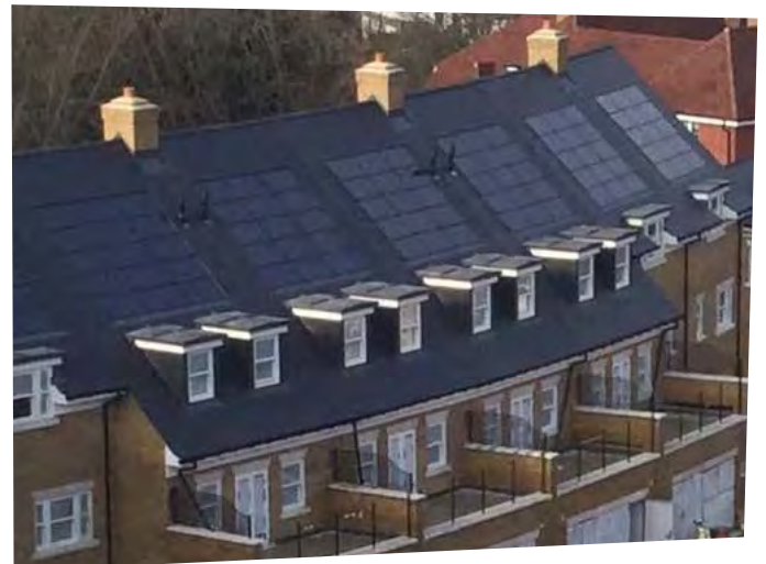
Demonstrating excellent standardisation of BIPV systems on adjacent homes.
