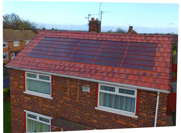
Colour matched 'in-roof solar' BIPV, where the colour of the solar panels has been matched to that of a modern terracotta roof tile on new build housing.
