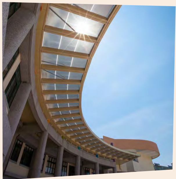
Clear solar glass, a second-generation technology, used as a canopy at a school building, Nantou, Taiwan.
