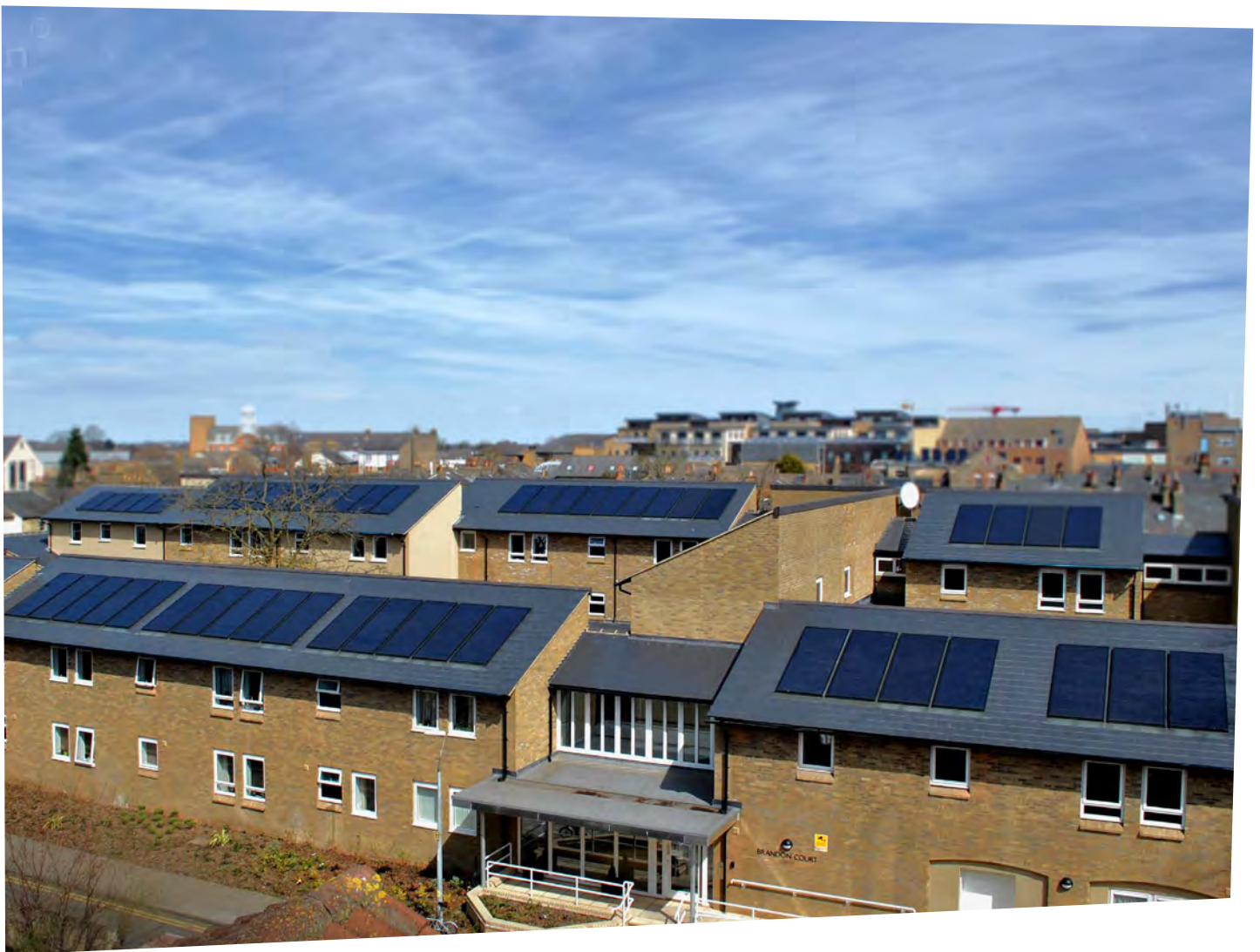
A 'broken block' approach to BIPV panel layout was used on this council-owned social housing refurbishment in Brandon Court, Cambridge.
