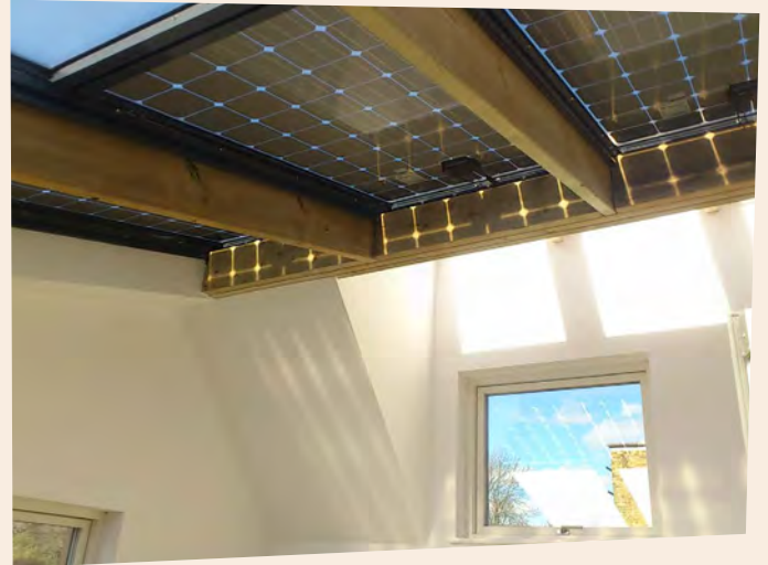
Monocrystalline glass-glass panels.
