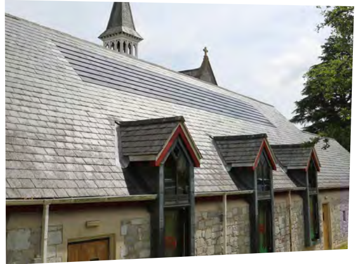
C21e solar slate has been used to integrate the solar system with the existing appearance of St Paul's Church in Devon, a grade 1 listed building (see the case studies section).
